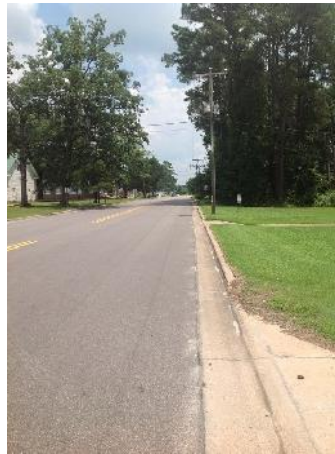
View looking down East Bear Grass Road showing existing wide lanes.
