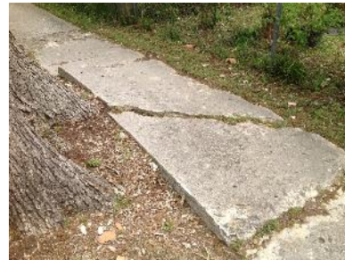
Damaged Sidewalk
