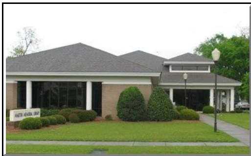
On October 2, 1995, the dream of a modern facility was realized when the new Martin Memorial Public Library was dedicated. Image Source: BHM Regional Library System.
