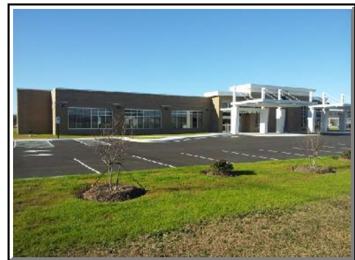
Metropolitan Community Health Services in Williamston, North Carolina. Image Source: A.R. Chesson Construction Co., Inc.
